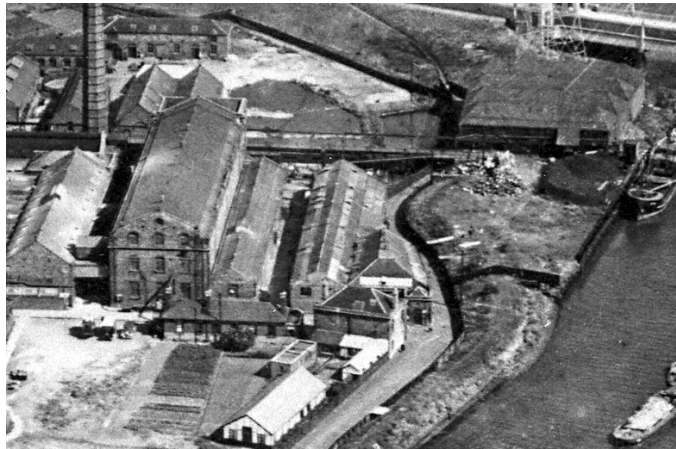
The jute warehouse to the left, reused as the William Warne rubber factory
